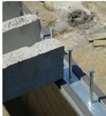
Clever Planks, showing rebates and steel studs that facilitated composite connection to steel beams
