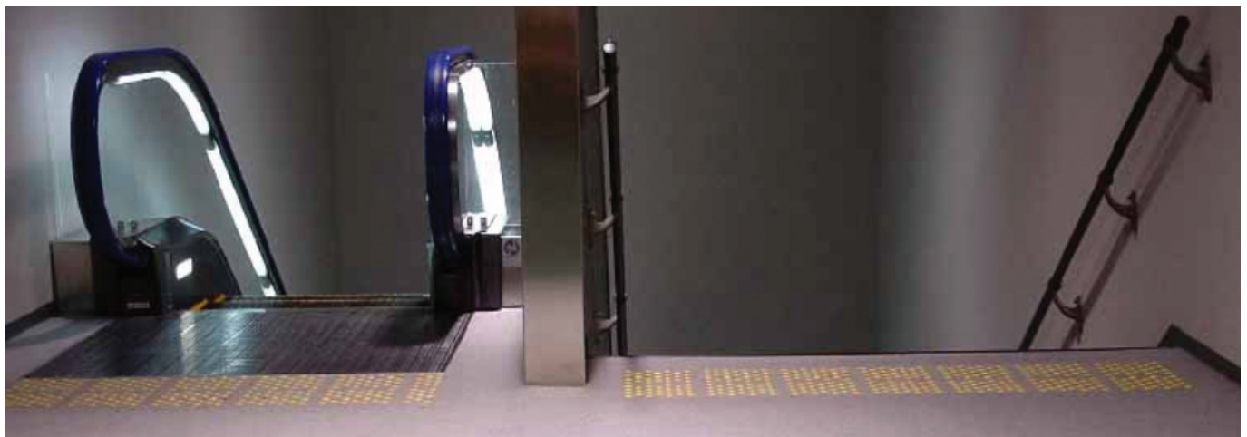
Raised tactile ground surface indicators
