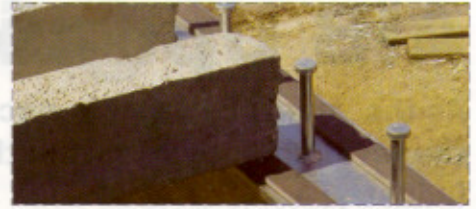
Close-up of clever plank connection prior to the application of topping concrete showing rebates, steel studs and steel beam
