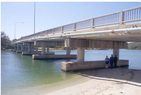
Photograph 1. General view of Bridge
