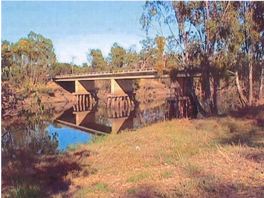
Photo 1. General view of Dawson River Bridge, Queensland
