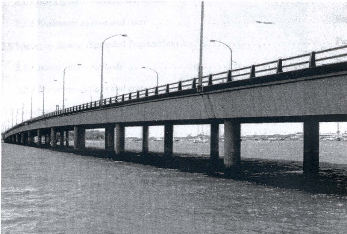
Photo 3. General view of Nerang River Bridge, Sundale, Queensland
