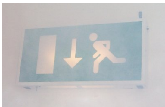
Figure 6.2 Smoke obscured exit system
