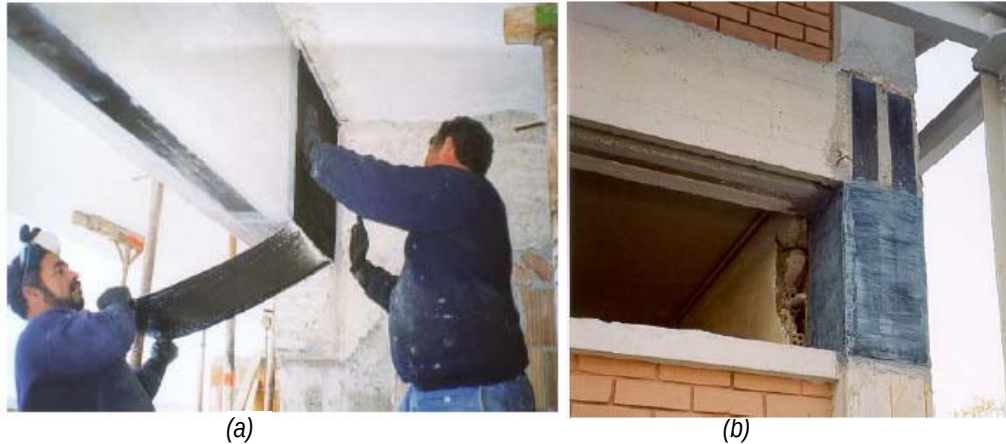
Figure 6-3: Schematic illustration of reinforced concrete element strengthened in shear with FRP: (a) FRP sheets or fabrics bonded to the web; (b) wrapped or U-shaped FRP (the concept shown in D is applicable to both beams and columns) (FIB Bulletin 14, 2001).
