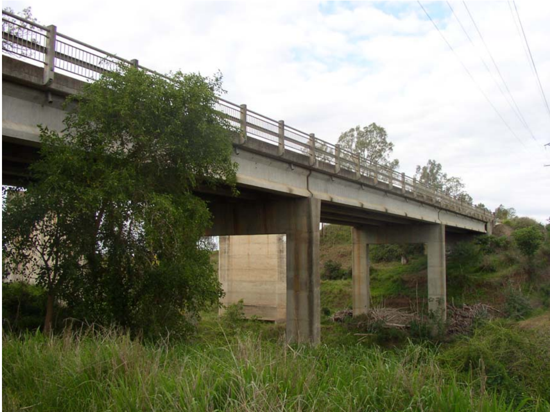
Figure 2-2 Photos of the Tenthill Bridge
