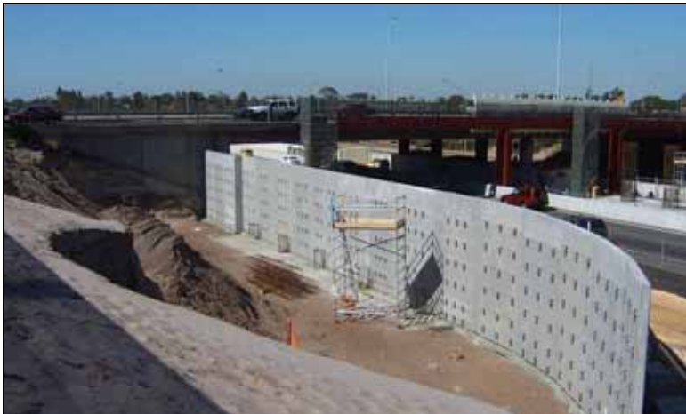
Figure 4.2: Leach Highway Bridge: Pre-cast concrete abutment walls
