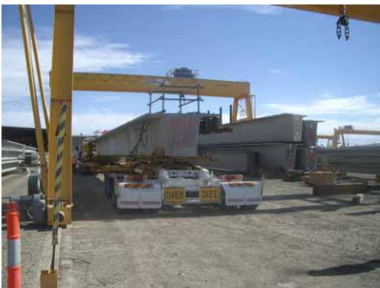
Figure 4.7: 'Jinkers' being loaded with post-tensioned bridge beams
