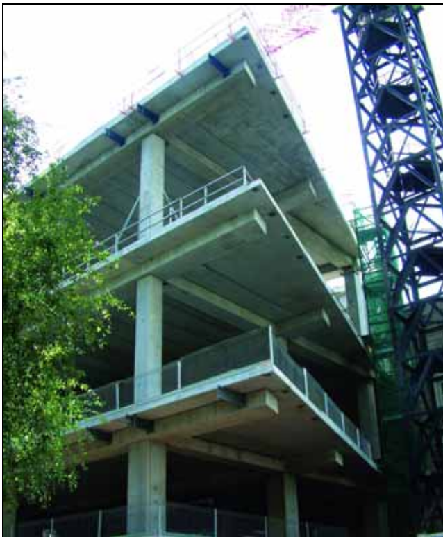
Figure 4.20: Example of a building using Hollowcore system.
