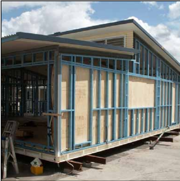
Figure 4.13: With completed roof in place the framework and fitting out commences.
