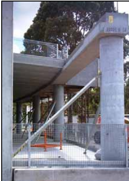
Figure 4.22: Hollowcore planks, beams and columns (showing support) onsite.
