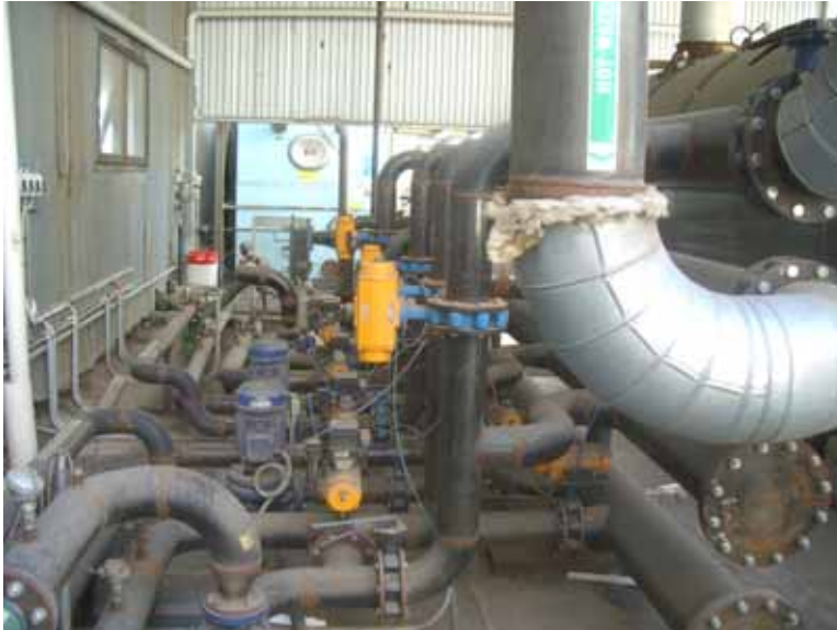
Figure 4.5: Boiler system used to accelerate curing of the moulded concrete.
