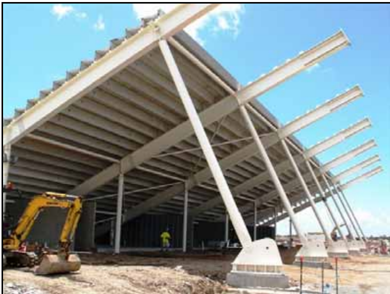
Figure 4.19: Steel structure and concrete plats onsite.
