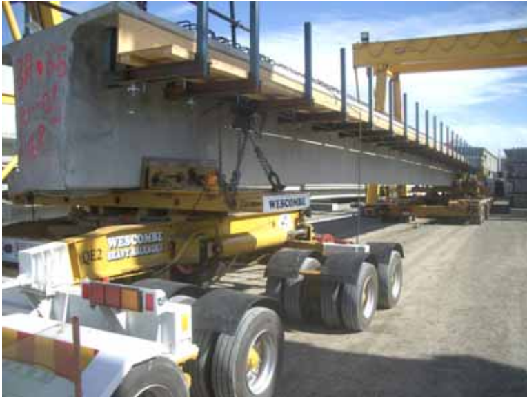
Figure 4.6: Safety rails fitted to beam and loaded onto 'jinker' for transportation.
