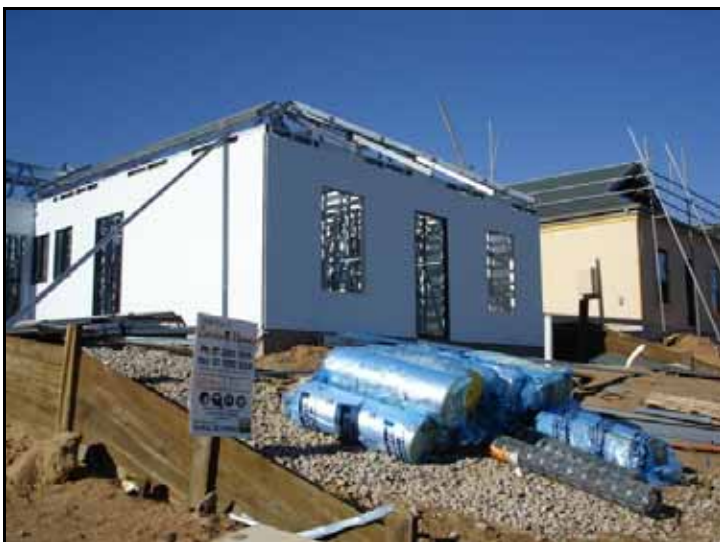
Figure 4.25: Construction onsite (Source: Monarch).
