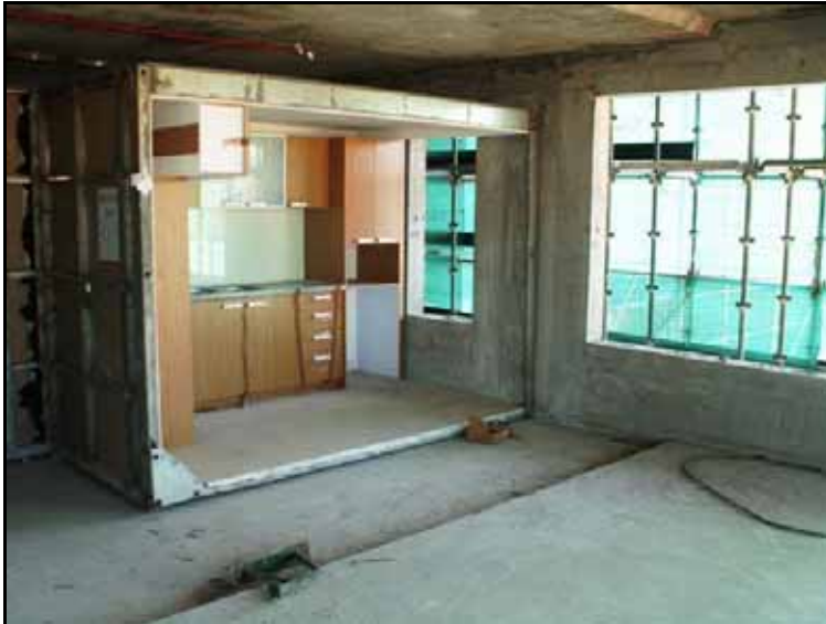
Figure 4.10: Kitchen module in place by window (note drop down floor).
