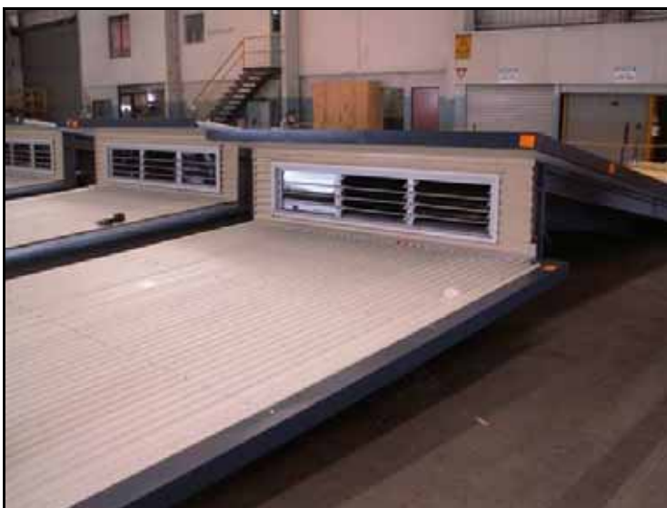
Figure 4.12: Completed roof sections assembled at ground level.
