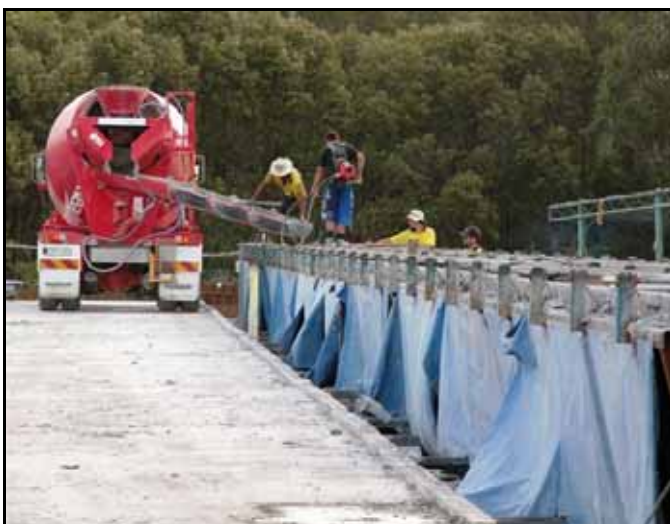
Figure 4.18: Pouring the concrete plats.
