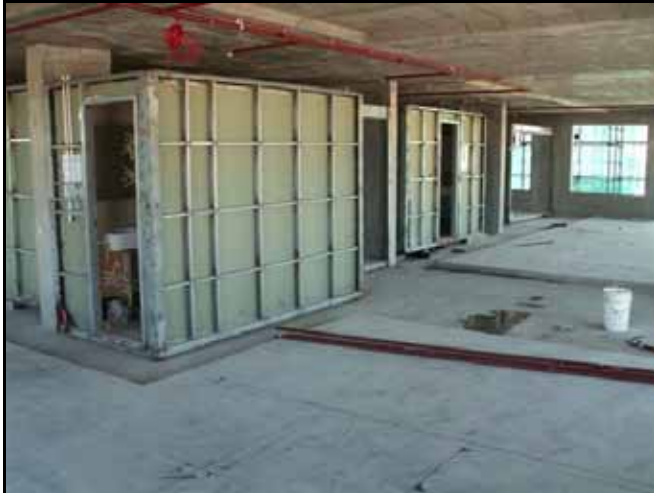
Figure 4.9: Modules in position (note void above for services).
