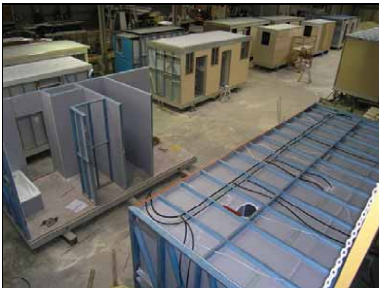
Figure 4.27: Bathroom modules in production (Source: Monarch).
