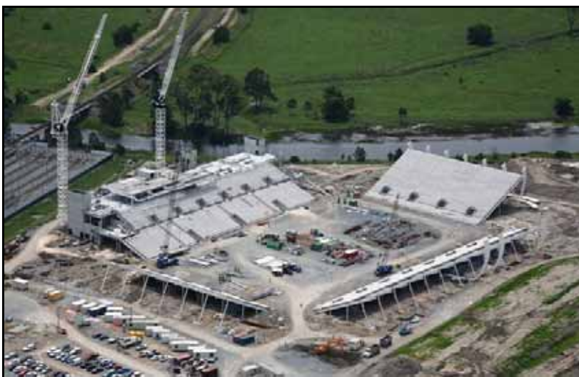
Figure 4.16: Robina Stadium site January 2007 (Source: Watpac Construction).
