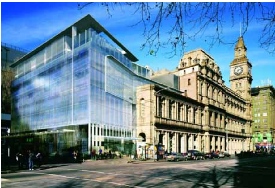
Figure 4.23: GPO Building Melbourne
