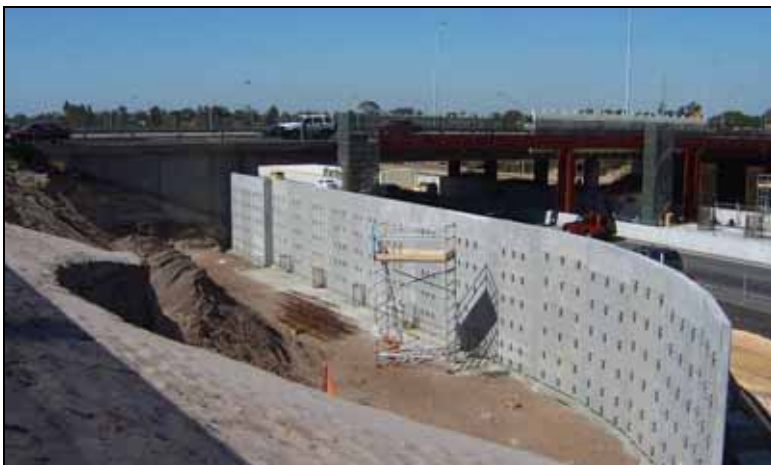
Figure 2.2: Leach Highway Bridge: Pre-cast concrete abutment walls
