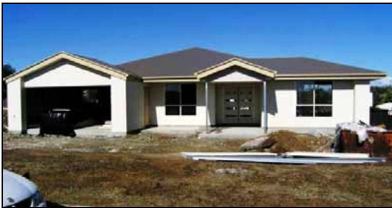
Figure 8.3: Completed house (Source: Monarch).
