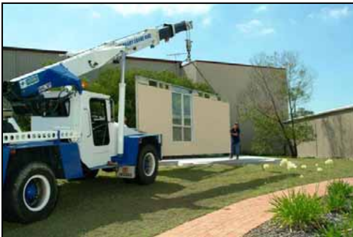
Figure 8.1: Lifting completed wall panels onto site (Source: Monarch).
