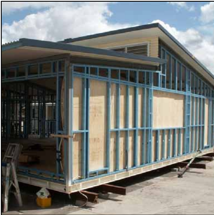
Figure 5.3: With completed roof in place the framework and fitting out commences.
