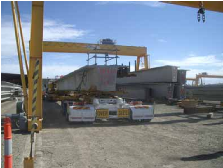
Figure 3.3: 'Jinkers' being loaded with post-tensioned bridge beams
