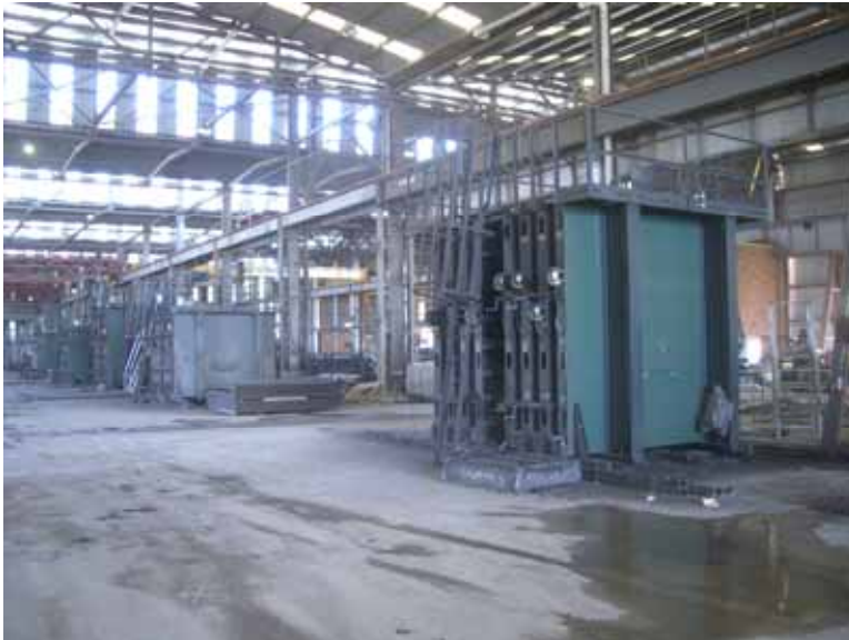
Figure 3.4: Vertical sound barrier moulds (Battery Moulds).
