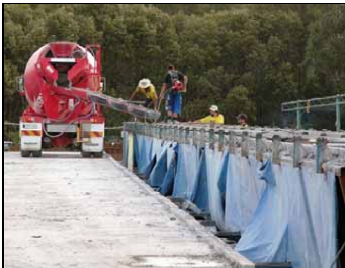
Figure 6.3: Pouring the concrete plats.
