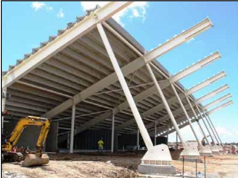
Figure 6.4: Steel structure and concrete plats onsite.
