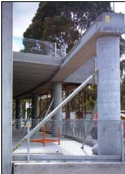
Figure 7.3: Hollowcore planks, beams and columns (showing support) onsite.
