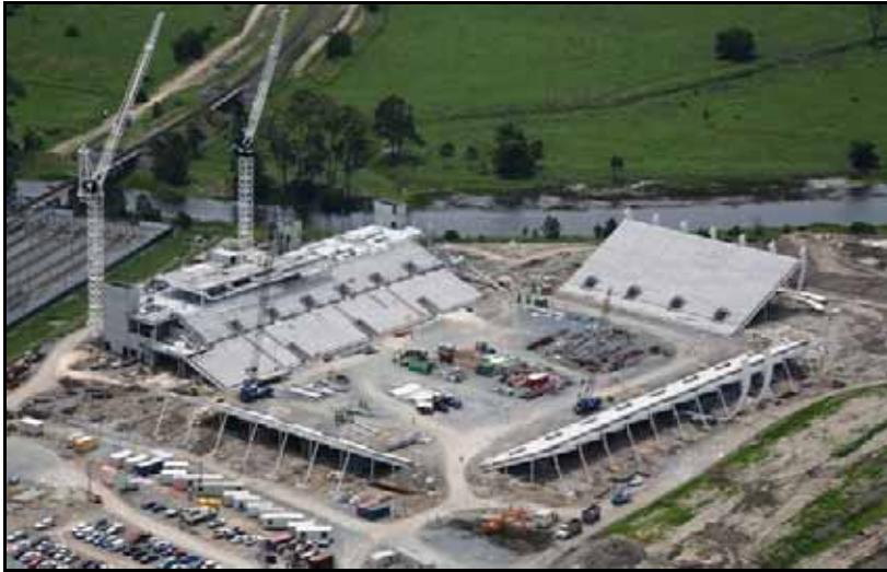
Figure 6.1: Robina Stadium site January 2007 (Source: Watpac Construction).
