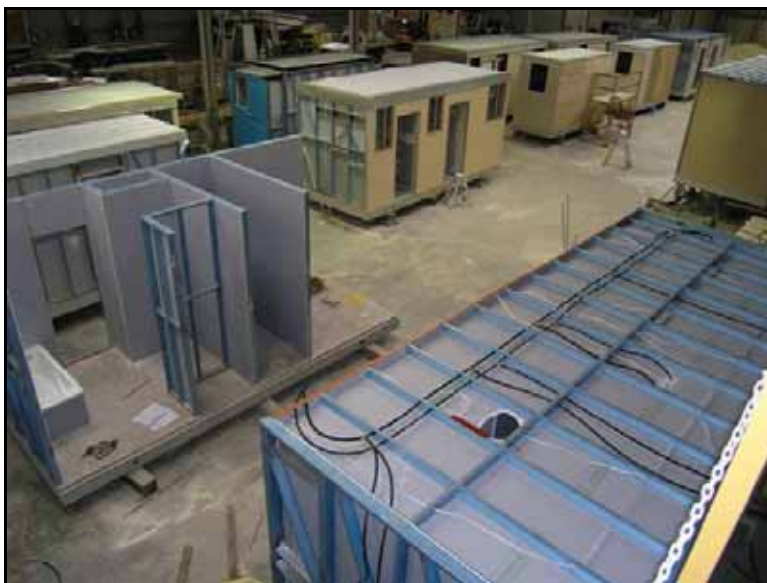
Figure 8.4: Bathroom modules in production (Source: Monarch).
