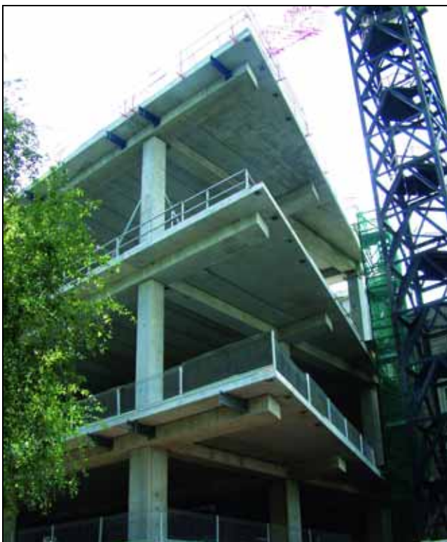
Figure 7.1: Example of a building using Hollowcore system.
