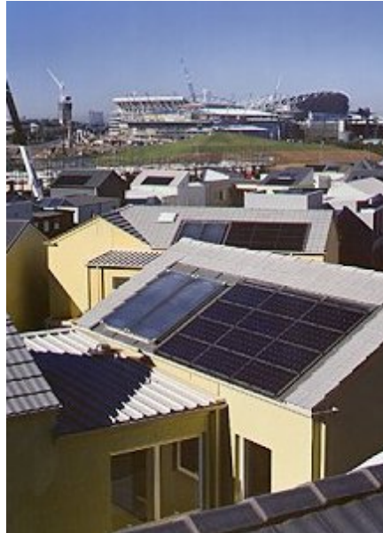
Figure 6.6 Partially integrated PV array at Newington
