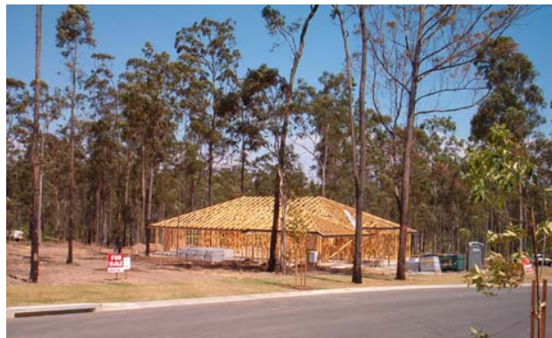
Figure 6.11 Sanctuary Pocket development under construction
