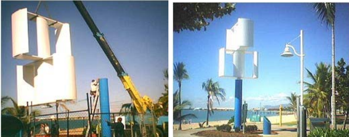
Figure 6.16 Installation of the Ropatec WRE.060 VAWT in Townsville
