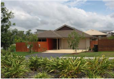
Case study 6, new (2005) dwelling, BV/C, good ventilation Images Author, 2006
