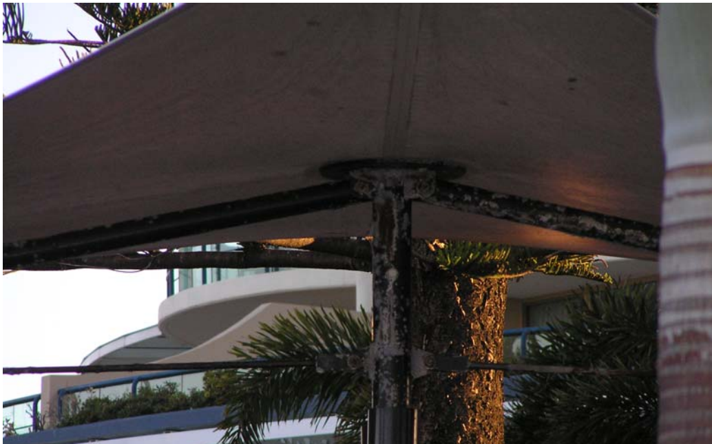
Figure 31. Canvas shelter with painted galvanised steel supports
