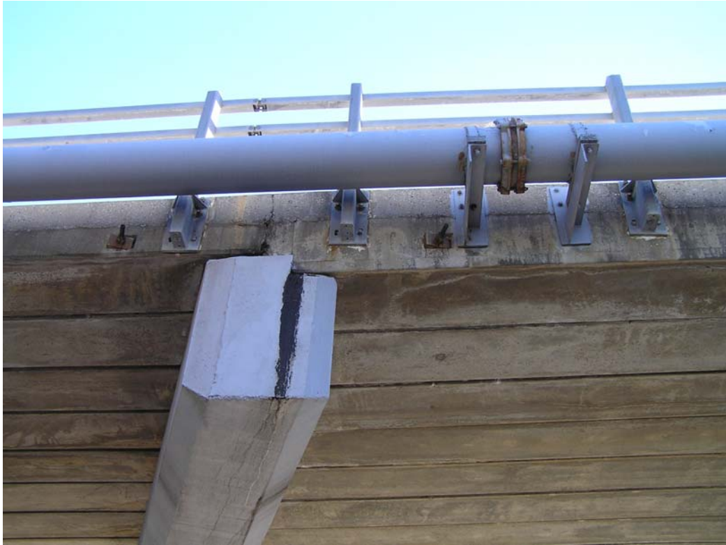
Figure 7. Pipeline and guard rail connections to bridge
