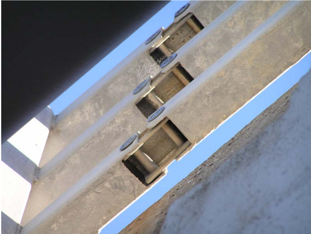
Figure 13. Underside of guard rails showing some signs of white corrosion product
