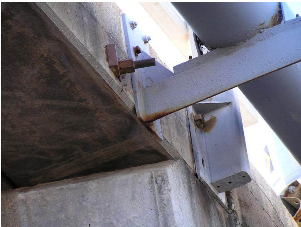
Figure 10. Pipeline and guard rail connections at northern end of bridge viewed from below
