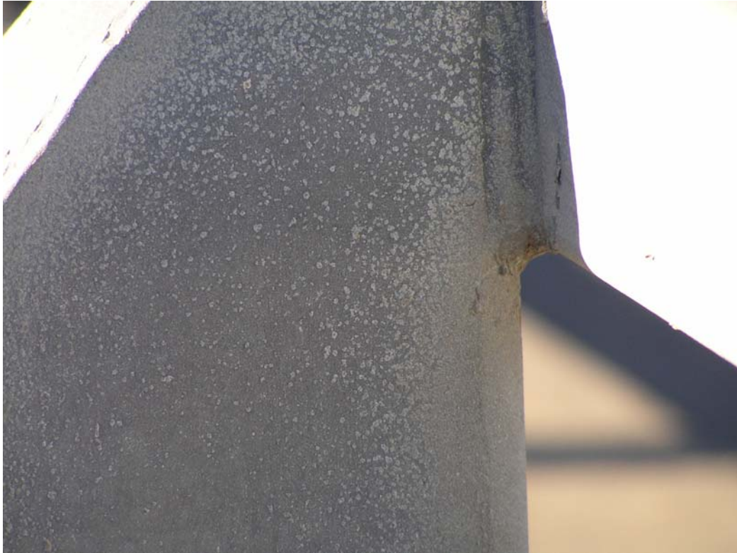
Figure 21. Close up of corrosion on guard rail
