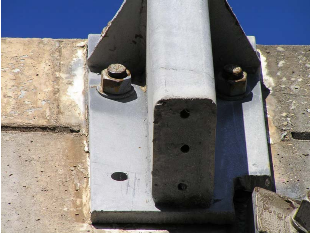
Figure 19. Guard rail support on western side of the bridge
