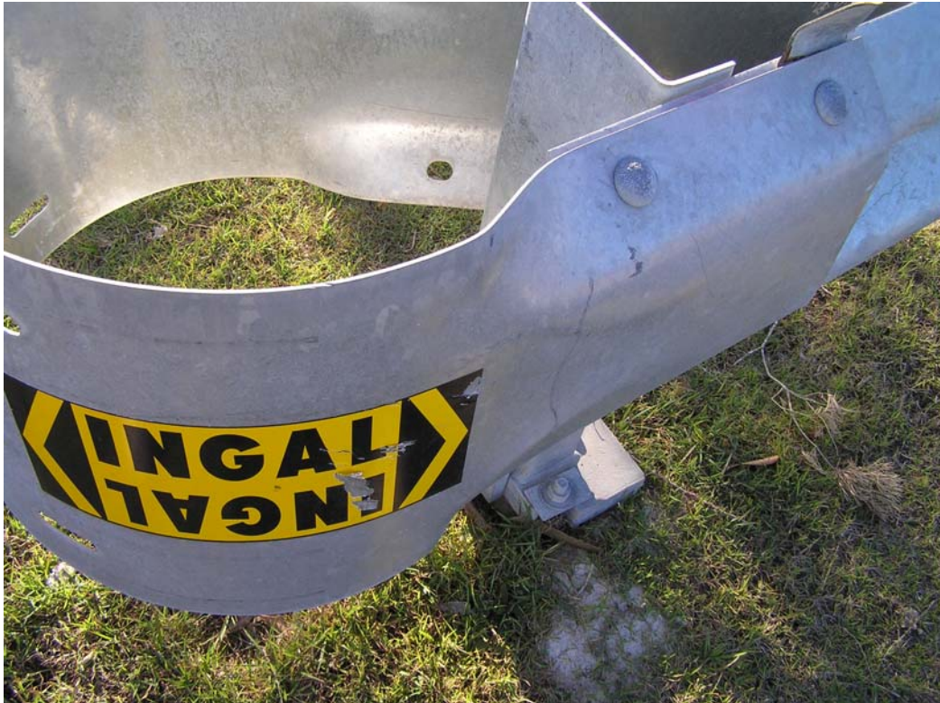
Figure 22. Galvanised crash barriers.
