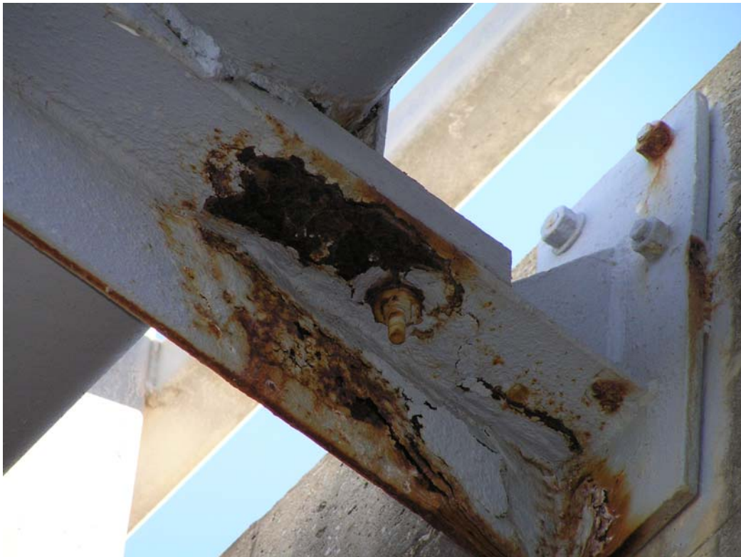
Figure 12. Pipeline support viewed from below showing red rust
