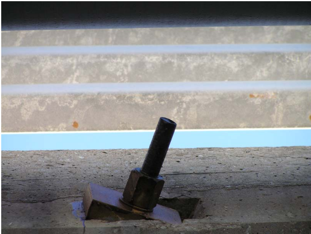
Figure 16. Guard rails seen from below showing white corrosion product and possible red rust
