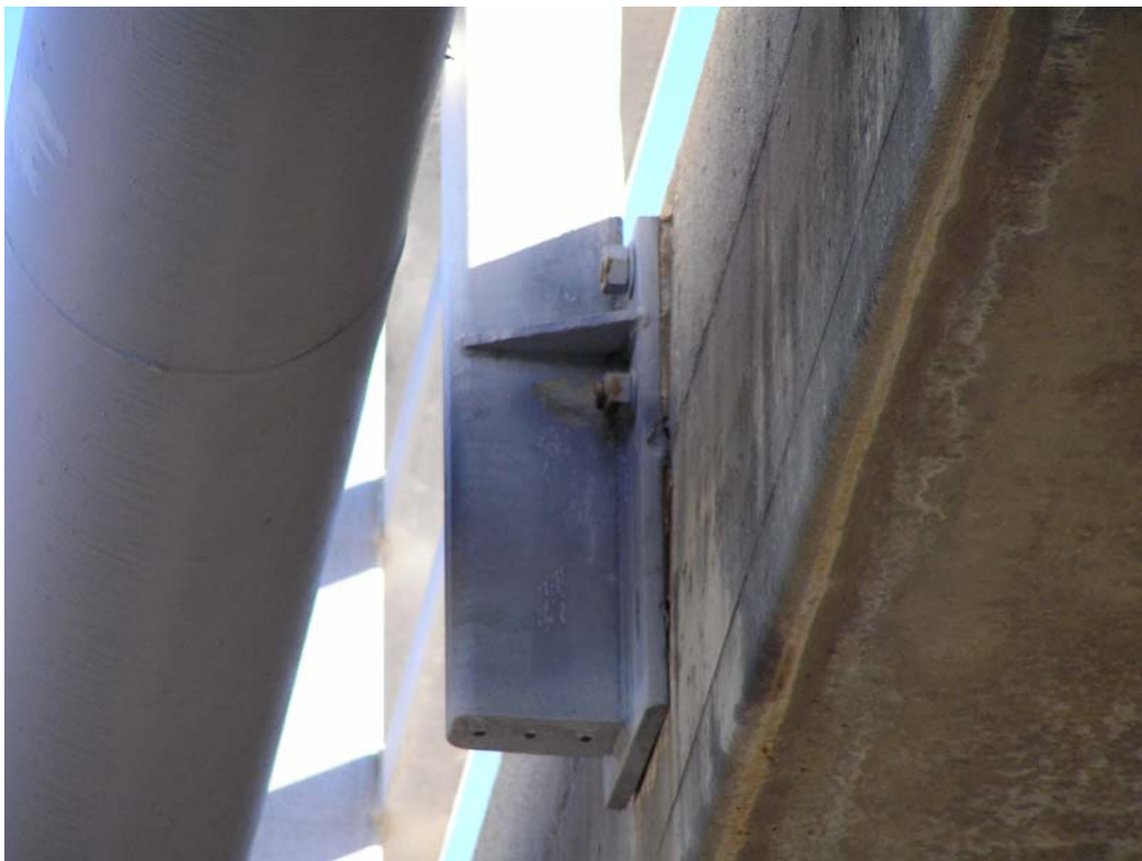
Figure 14. Guard rail support seen from below
