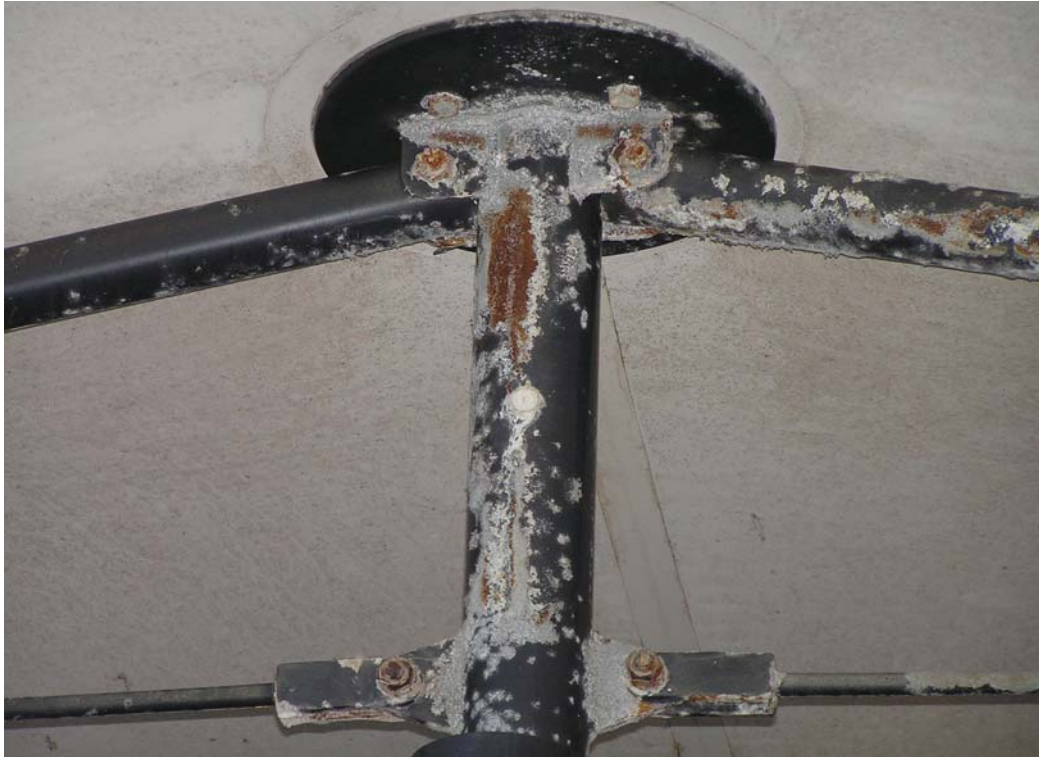
Figure 32. Close-up of shelter support showing red rust, white corrosion product and paint deterioration.
