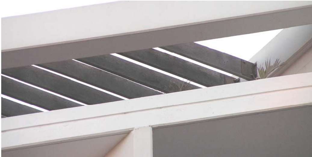
Figure 34. Galvanised Purlins on top floor of building showing white corrosion product
