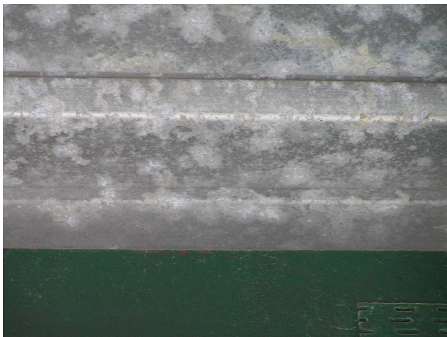
Figure 8 Close up of inside of roof sheeting of covered games area showing significant white corrosion product and some red rust.
