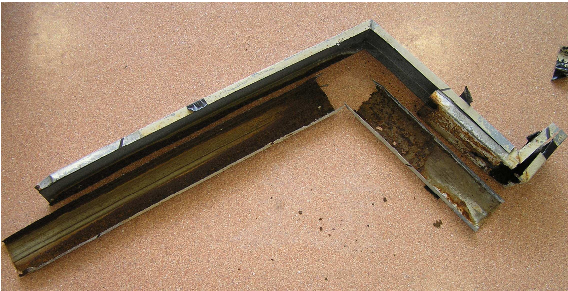
Figure A9, Inside of downpipe
