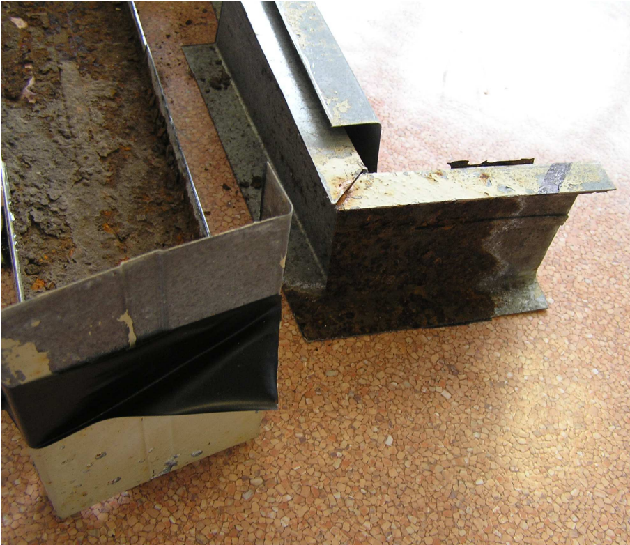
Figure A7, very top section of downpipe
