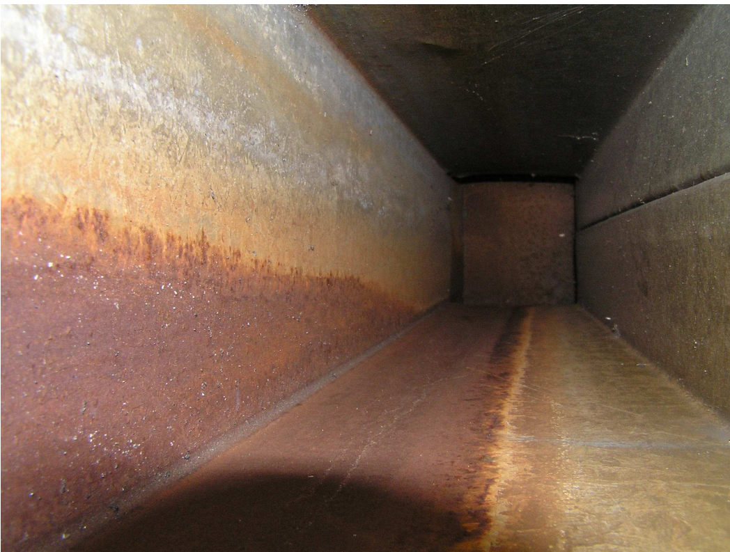
Figure A17, from inspection opening looking down
