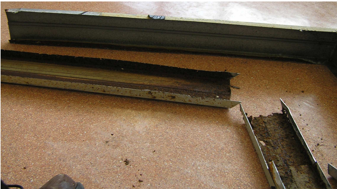
Figure A10, lower section of the downpipe
