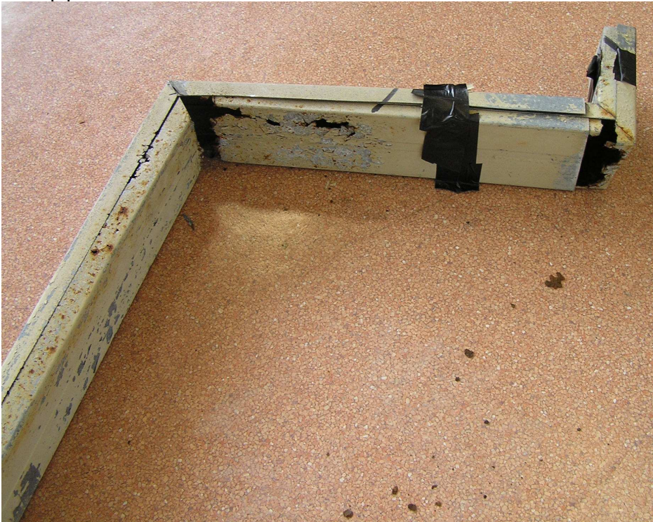
Figure A8, Top section of downpipe
