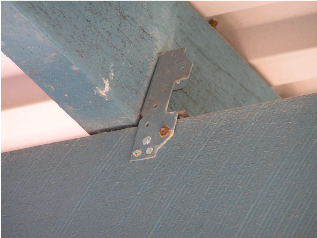
Figure 16 Triple grips on structure of covered set down showing signs of deterioration and roof fastener shank to red rust.
