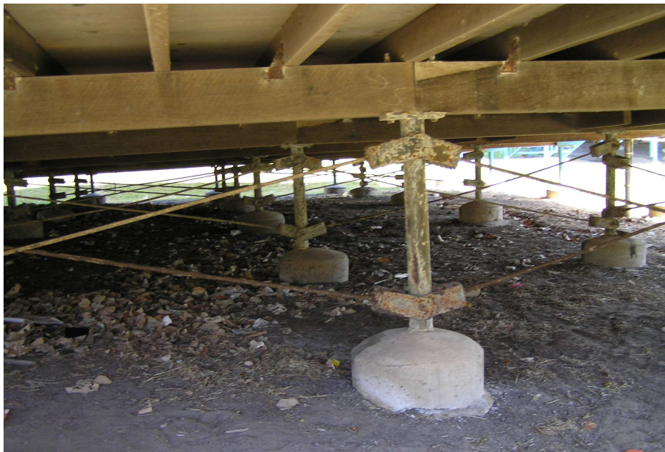
Figure 28. Significant deterioration of sub-floor metallic components on modular classroom.
