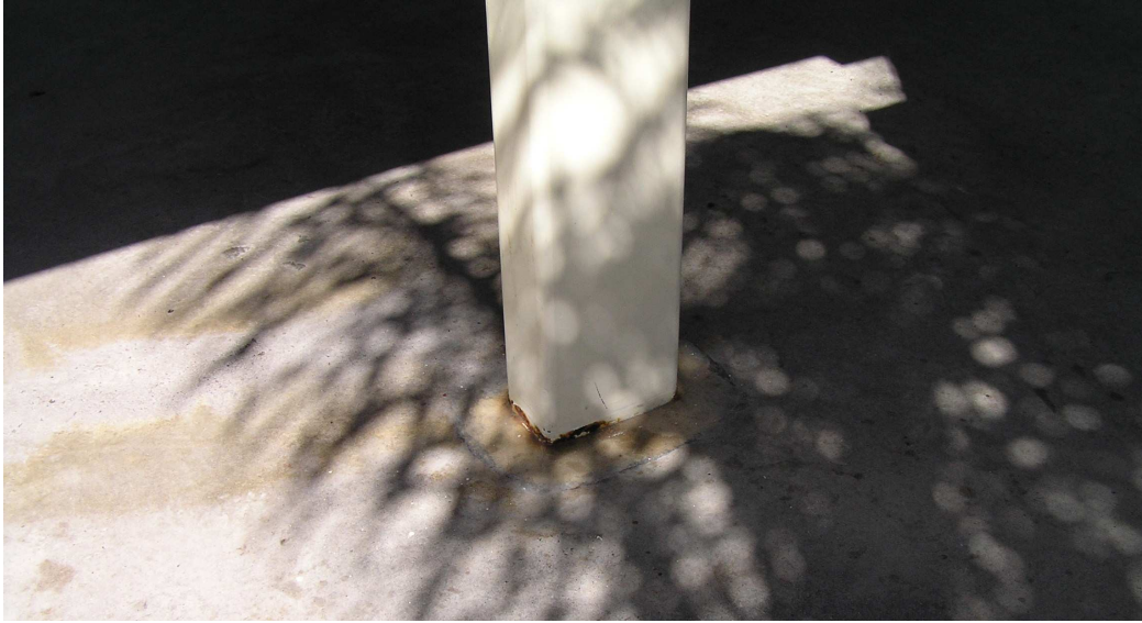
Figure 25 Footing of steel support showing red corrosion product.
