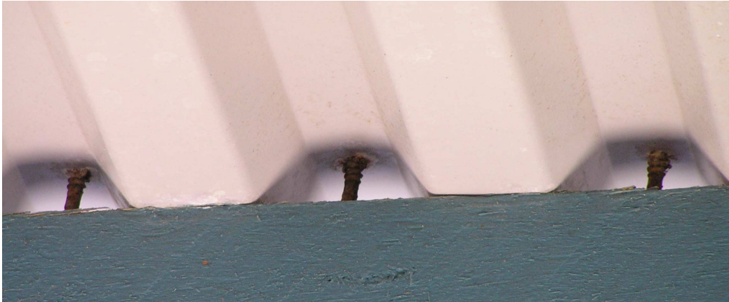
Figure 11 Covered walkway, fastener shanks are red rust and undercutting seen on Colorbond® sheeting.
