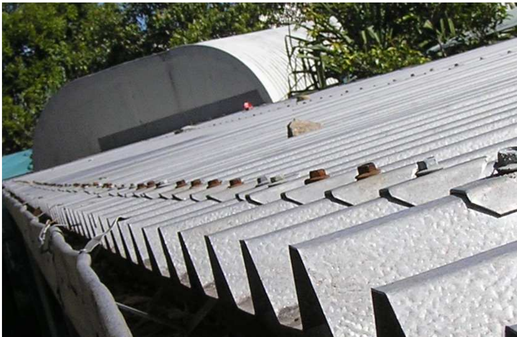
Figure 10 Roof fasteners showing red rust and white corrosion product.
