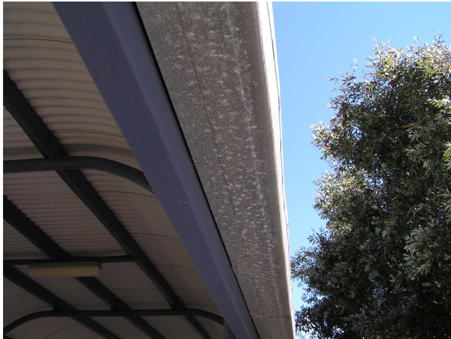
Figure 1 Underside of gutter showing significant corrosion.
