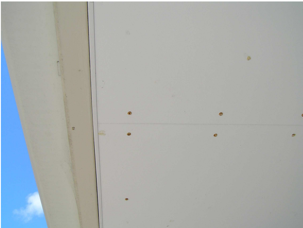
Figure 14 Fasteners in sheeting on porch.
