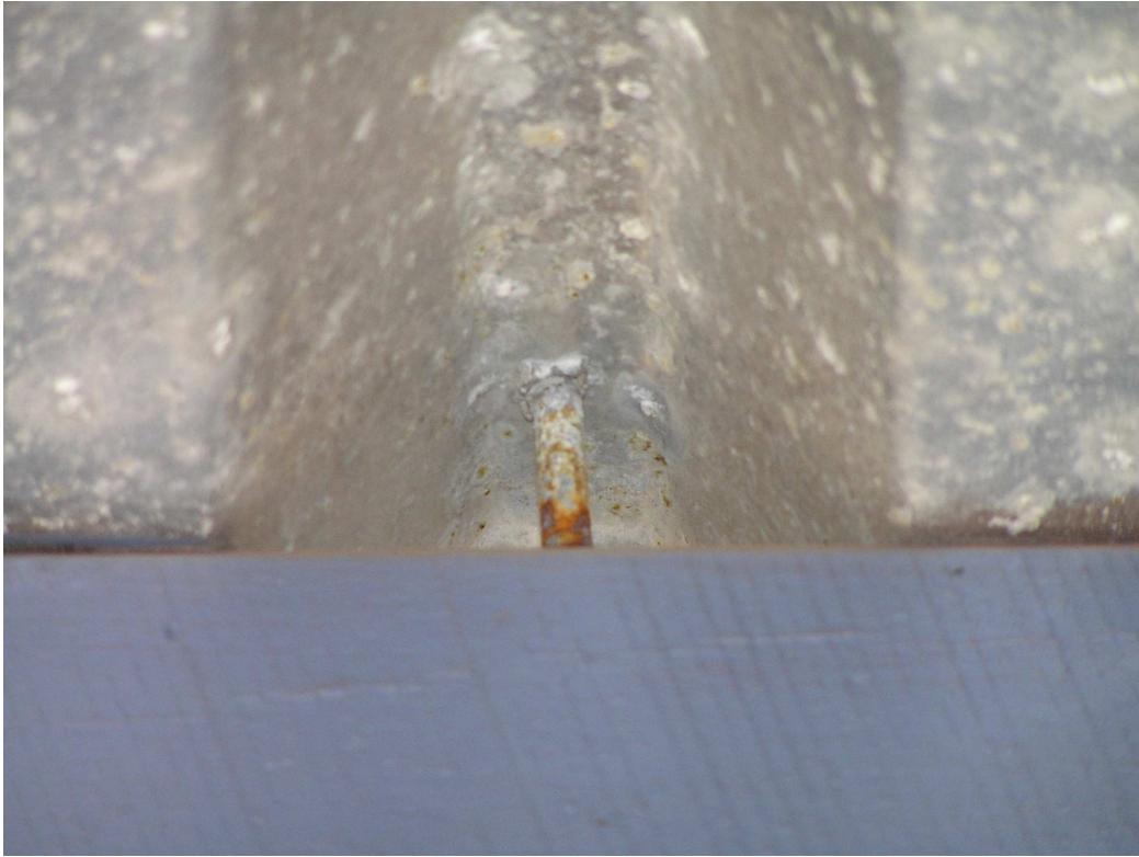
Figure 13 Heavily corroded fastener in sheeting of covered walkway.
