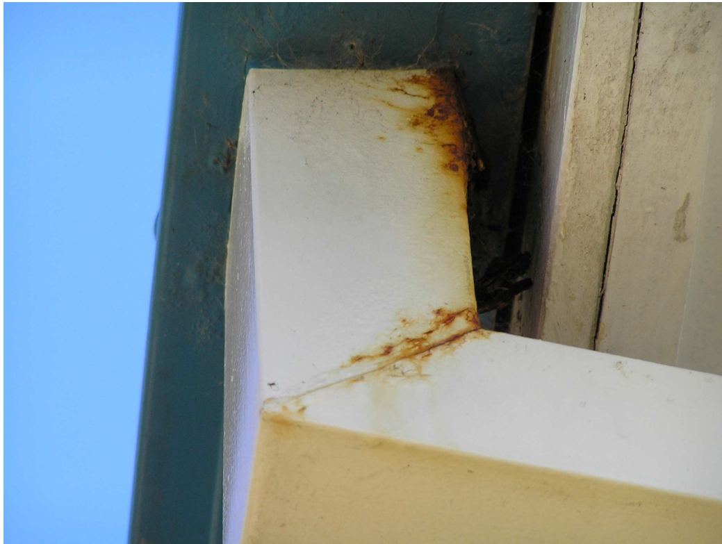
Figure 5 Rusting and deterioration on downpipe on modular classroom showing that problems are associated with the joints.
