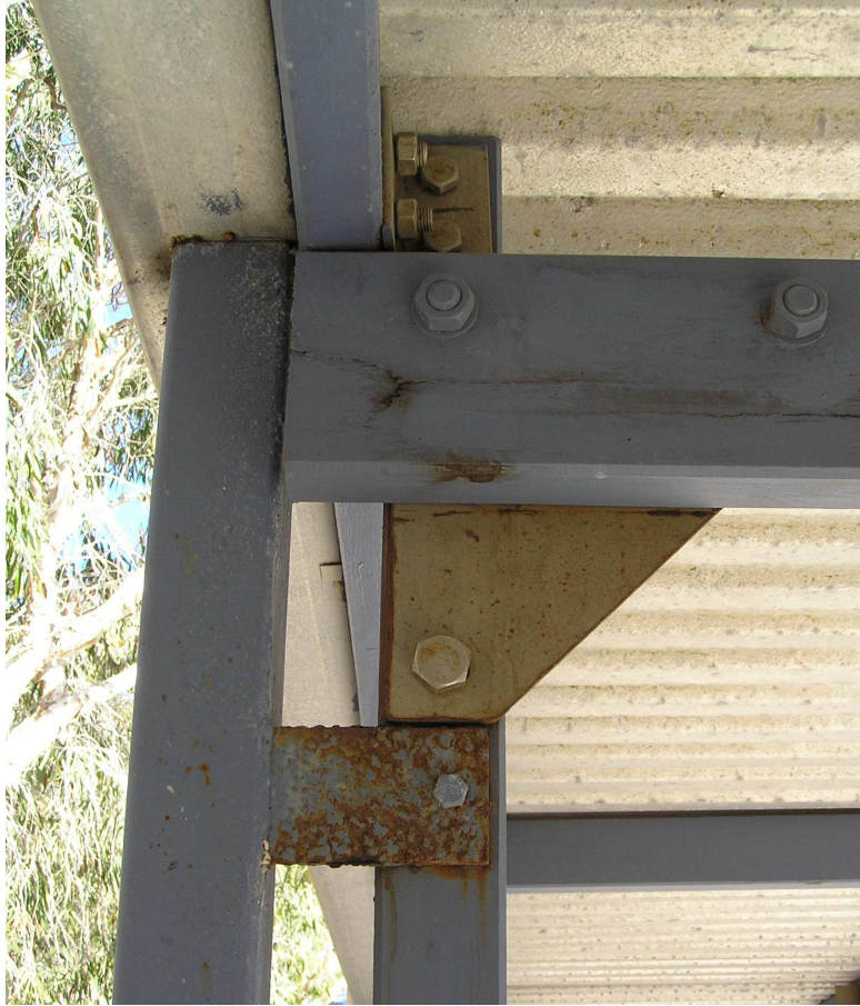
Figure 7 Top of downpipe also showing rusting of bracket from downpipe to support and stainless steel plates on walkway beams.
