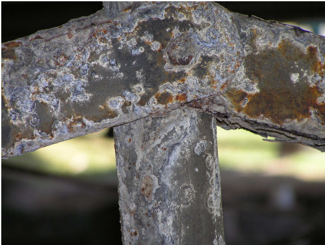
Figure 29 Two views of the corroding stump support of a modular classroom.
