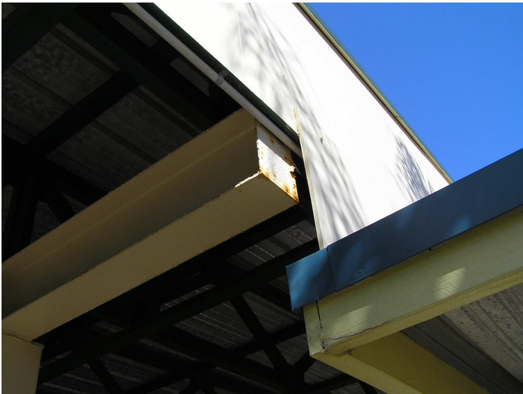
Figure 26 End of steel beam showing red rust break through.
