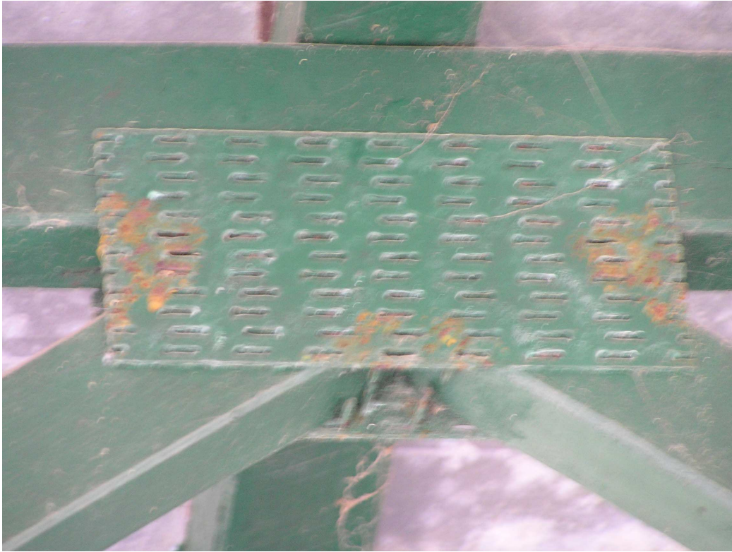
Figure 31 Close up of gang nail plates on inside of covered games area.
