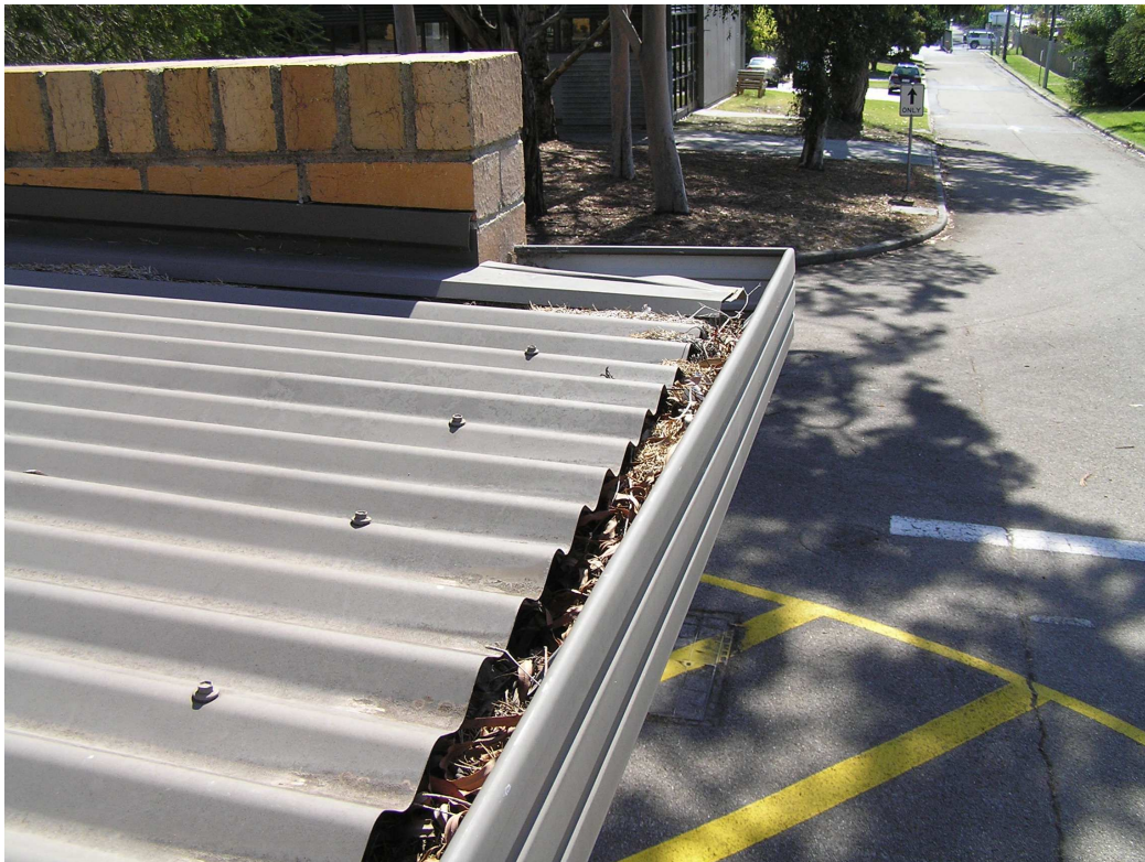
Figure 21, Flashing between wall and roof.
