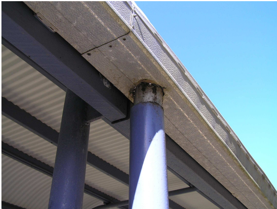
Figure 4 Deterioration around joint between gutter and downpipe (note loss of rivet heads).
