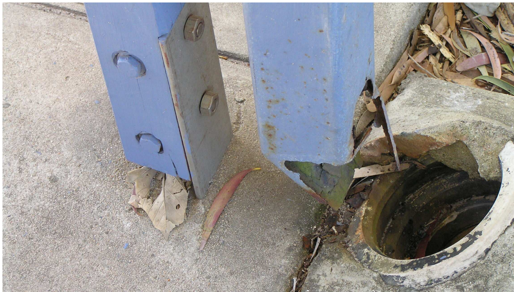
Figure 6 Bottom of square downpipe, steel completely rusted away.
