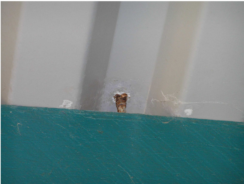
Figure 12 Corroded fastener under covered area, sheeting also showing undercutting.
