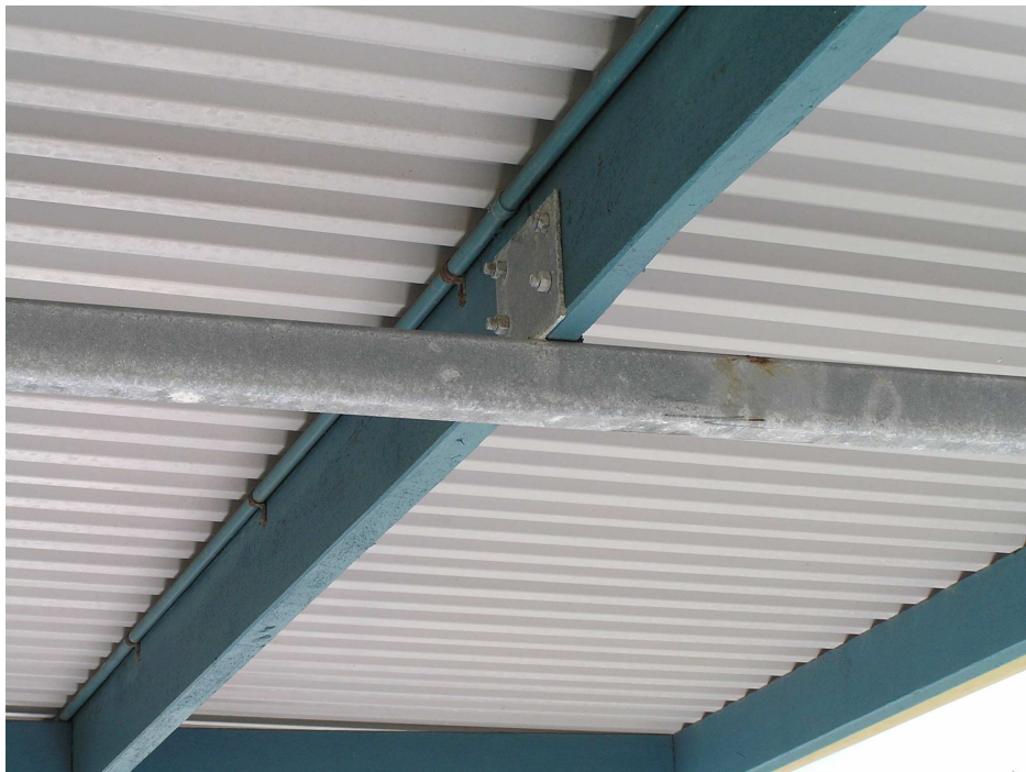
Figure 24 Covered walkway showing corrosion of galvanised support.
