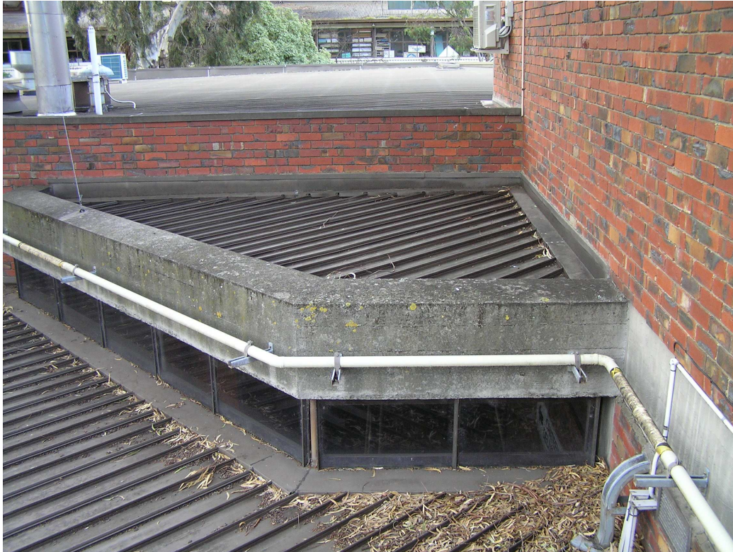
Figure 22. Flashing between wall and roof.
