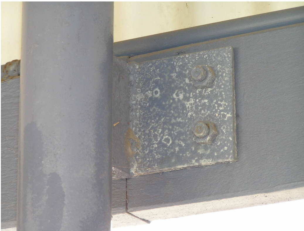
Figure 18 White corrosion product on painted steel brackets.
