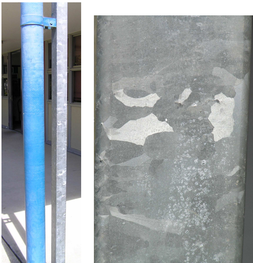
Figure 27. Galvanised post (right) and close up (left) showing signs of white corrosion product.
