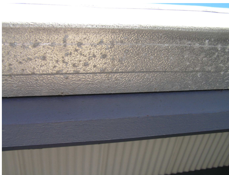
Figure 2 Underside of gutters (example of sheltered corrosion).
