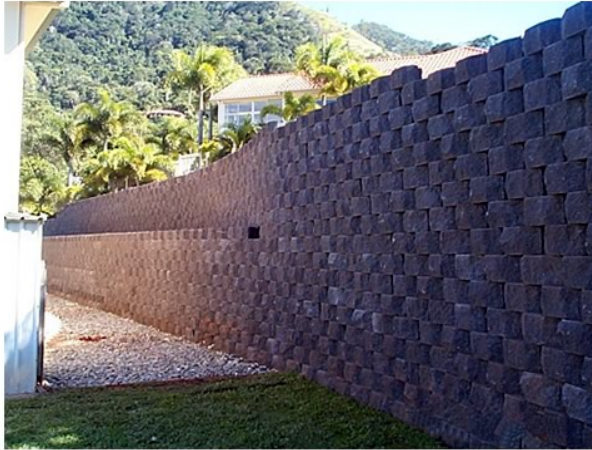
Figure 5: Typical retaining wall at a typical subdivision: blocking window level breeze.
