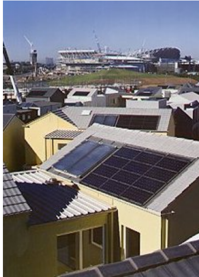
Figure 6.6 Partially integrated PV array at Newington
