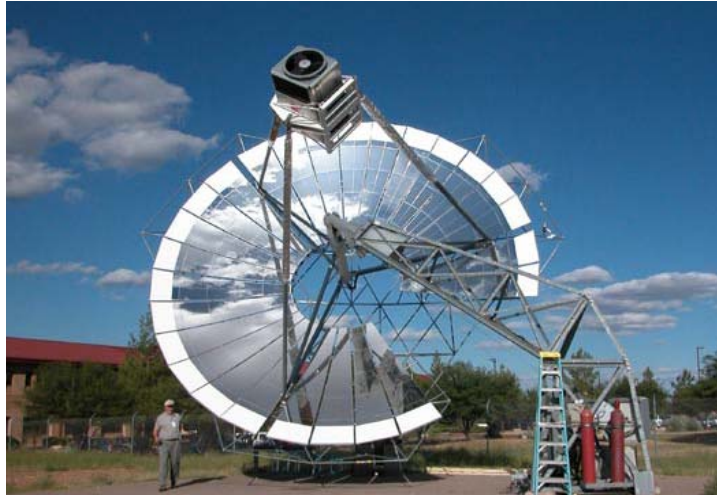
Figure 6.7 Stirling parabolic dish at Arizona Solar Centre
