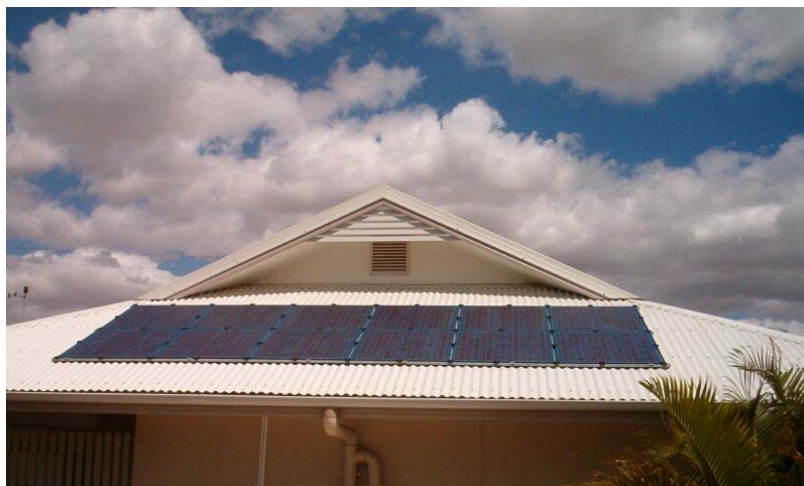
Figure 6.4 Traditional PV panels on the Rockhampton research house
