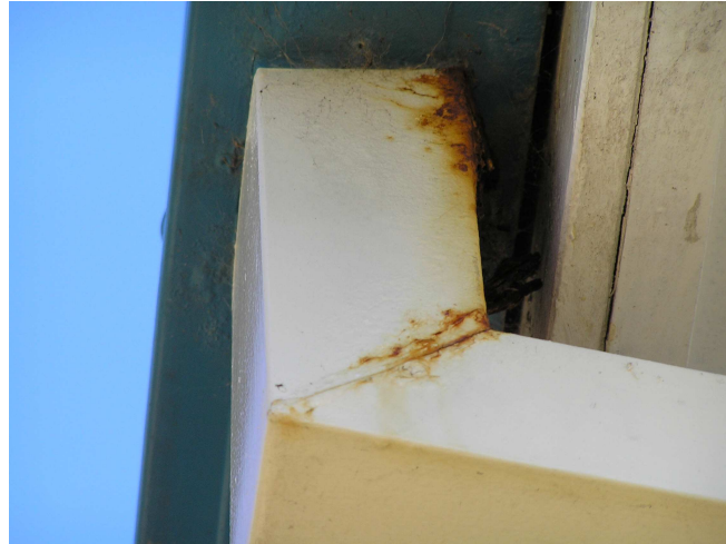
Figure 3.5 Rusting and deterioration on downpipe showing that problems are commonly associated with the joints.
