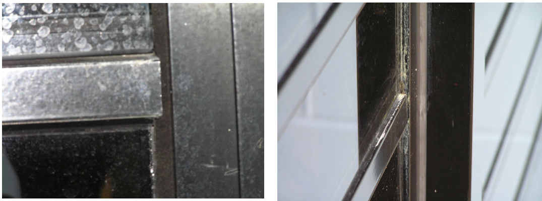
Figure 3.17. Example of metal window frames.
