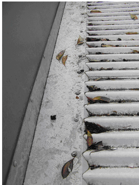
Figure 3.16. Flashing between wall and roof.
