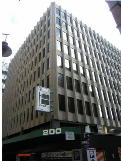
Figure 6.2 Exterior of CH1 building
