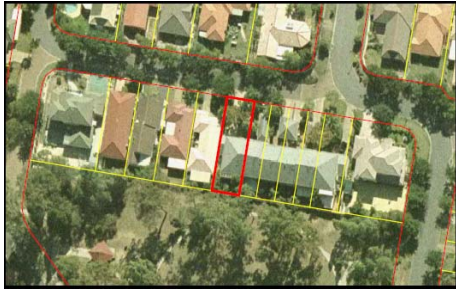
Figure 4-3 Aerial view of case study lots
