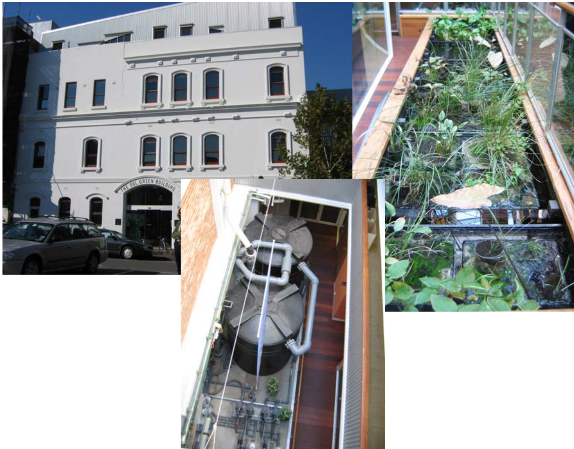
Figure 40: 60L Building facade, rainwater storage and treatment (centre) and reclaimed water feature
