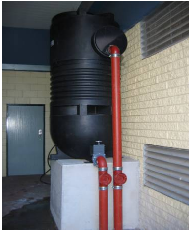
Figure 35: Atherton Gardens greywater treatment, CDS screen and subsurface wetland
