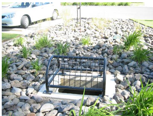
Figure 14: Weir to stormwater gross pollutant trap
