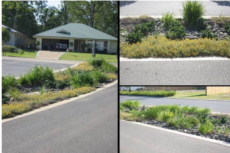
Figure 16: Swales with rocks and native vegetation for stormwater management.
