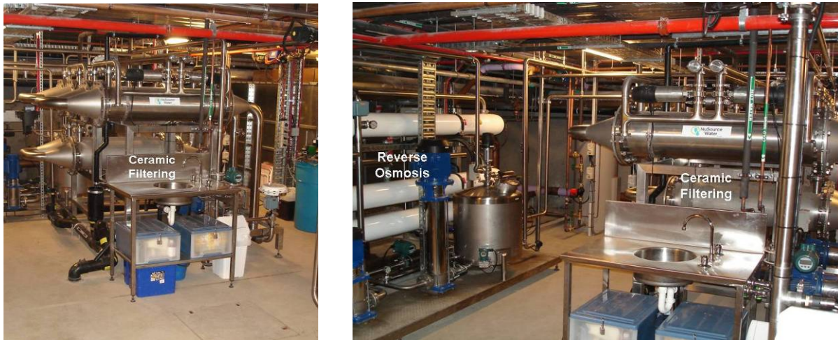
Figure 24: Multiwater treatment plant at CH 2 building
