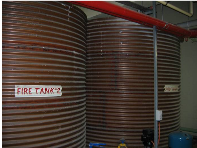
Figure 32: Atherton Garden fire tanks used for rainwater storage
