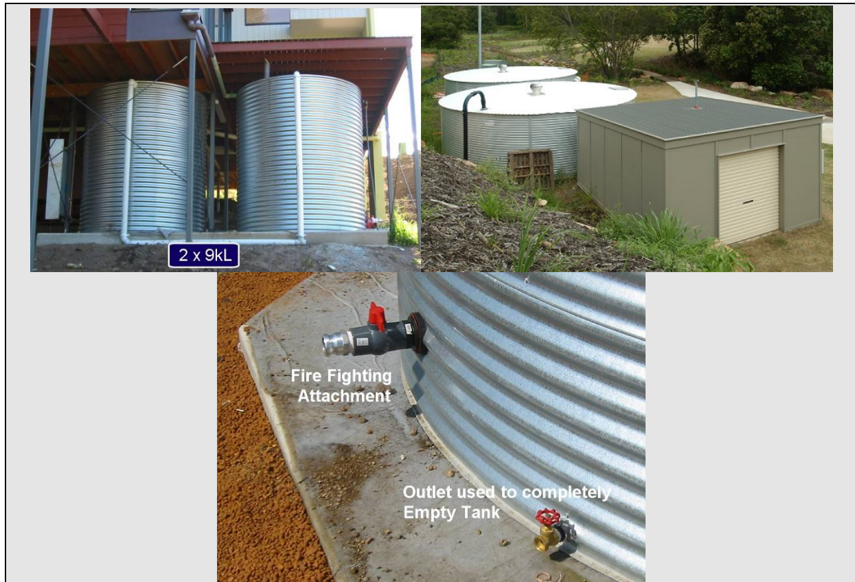
Figure 20: Household raintanks, stormwater tanks and outlets at Payne Road
