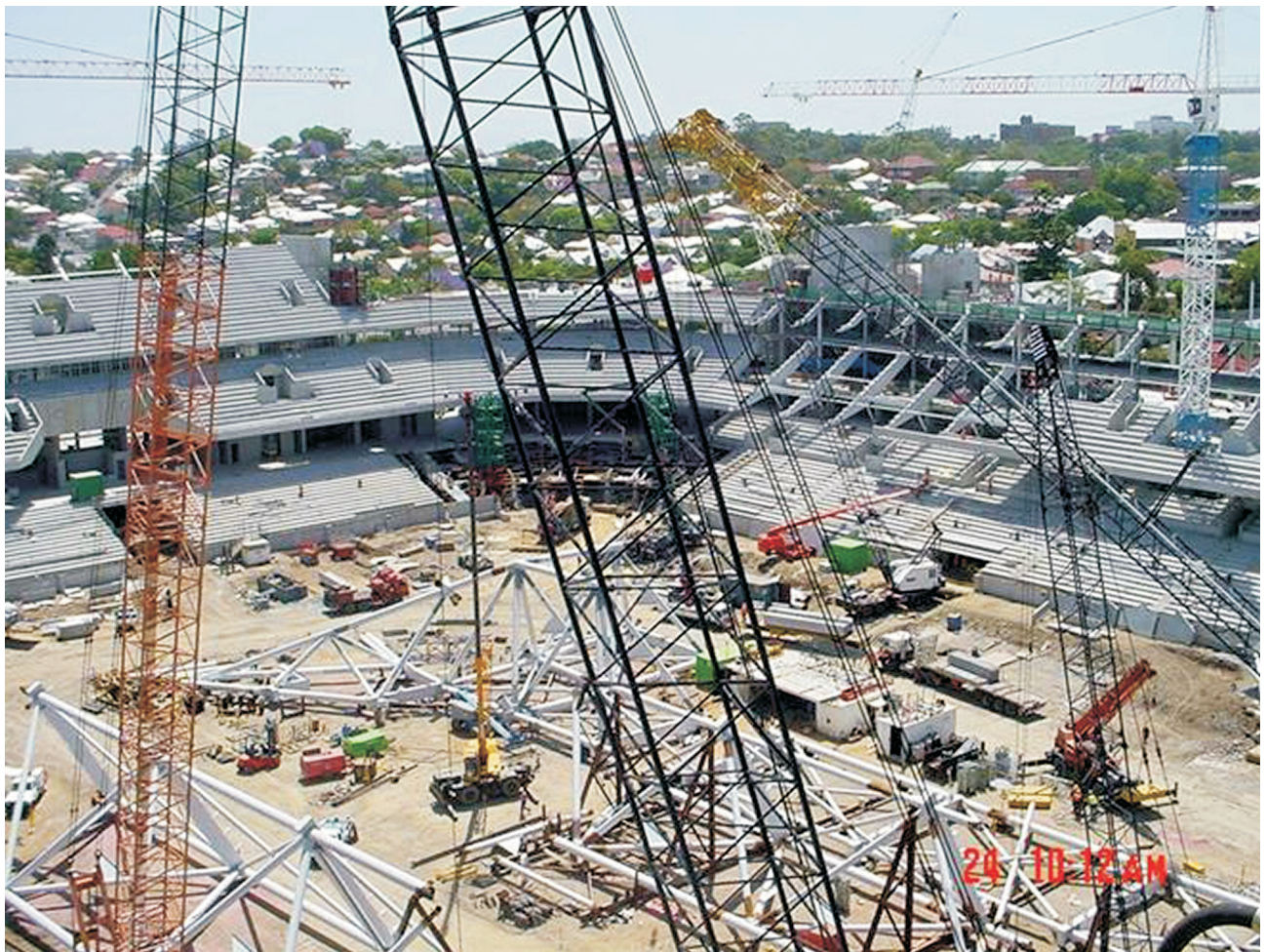
Figure 4: Stadium under construction (Source S. Davies, Arup)
