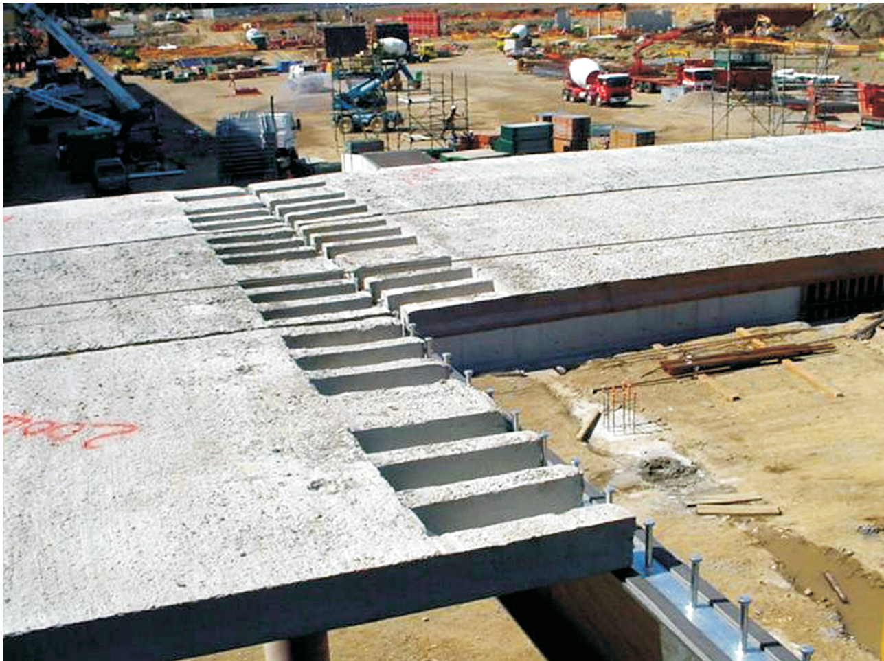
Figure 3: Precast planks being placed ready for composite connection (Source S. Davies, Arup)
