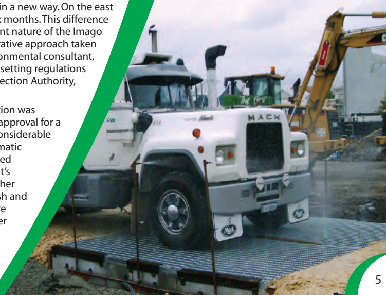
Wheel wash in use
