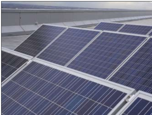
50 Lonsdale St Melbourne features solar panels for tempered hot water for showers. © Erica Lauthier, courtesy DEWR.
