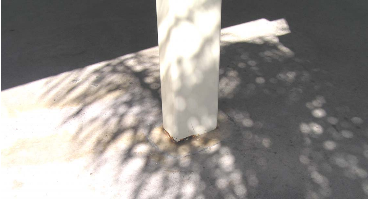
Footing of steel support showing red corrosion product
