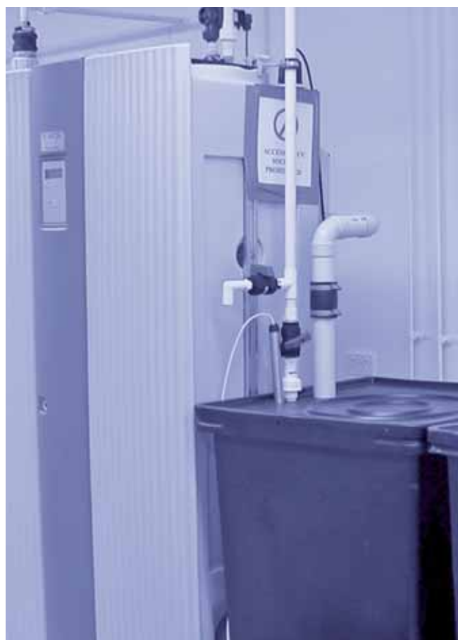
Greywater system — Pontos Aquacycle
