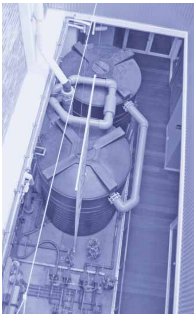
Rainwater collection system — 60L
