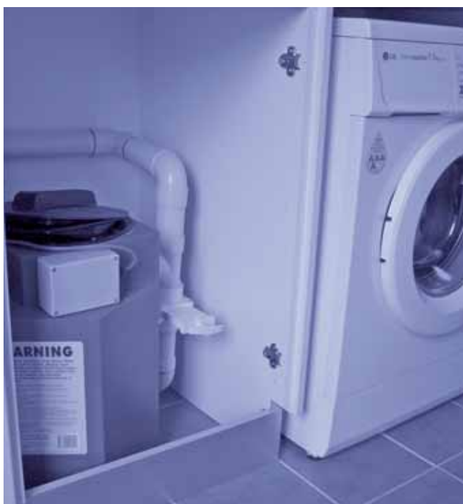
Greywater system — Ecocare diverter
