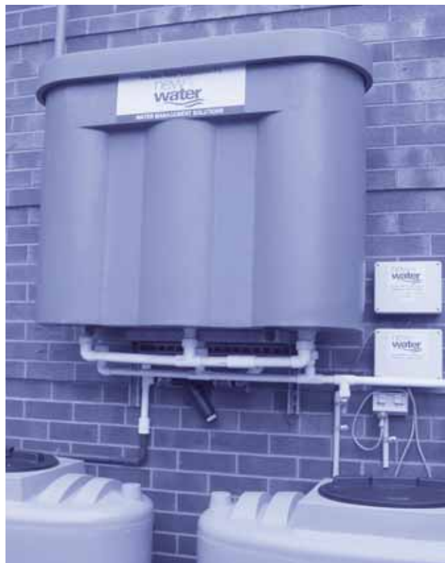
Greywater system — New Water
