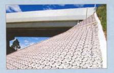
The pre-cast concrete blocks made up of two components: a 'lock block' and a 'key block'. The male and female parts of these blocks link together in an infinitely repeating pattern providing multi-dimensional stability and integrity over large areas. This feature, as well as enhancing the hydraulic characteristics, prevents major revetment failure.
