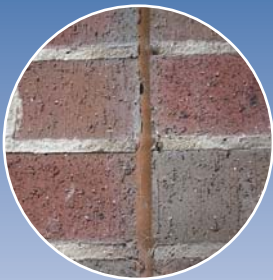
Traditional foam & mastic
