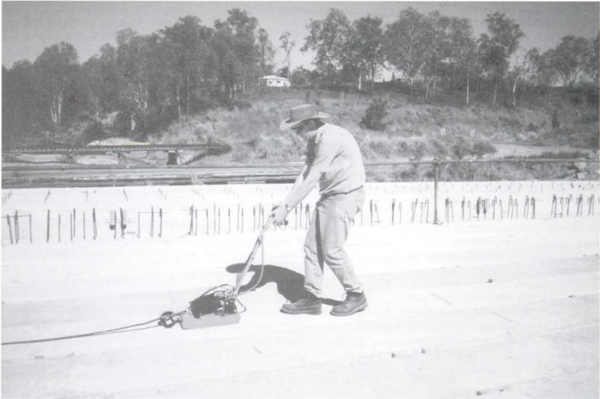
Ground penetrating radar was able to provide accurate images of internal defects in deck beams of the Cattle Creek Bridge, to within five millimetres.
