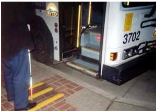
Figure 4.3 Detectable directional guidance surface
