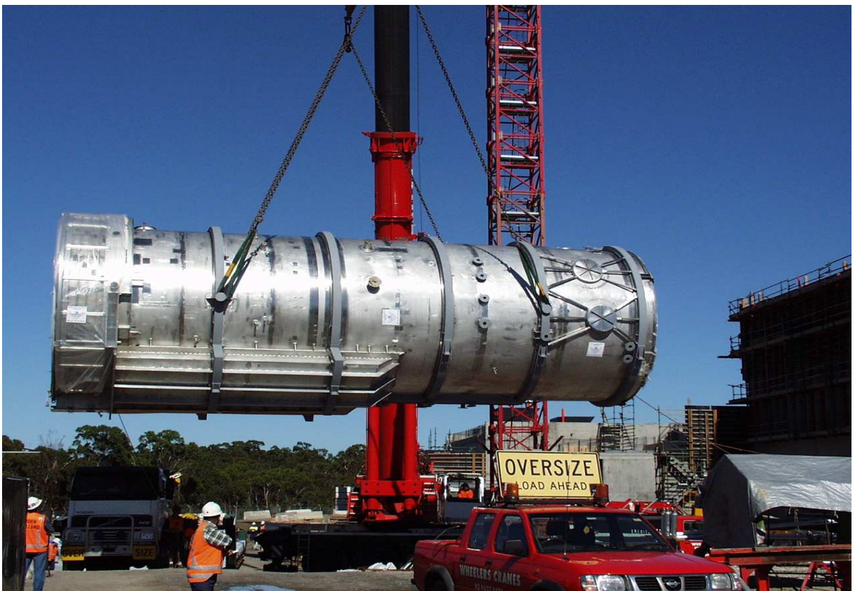
Replacement Research Reactor, Lucas Heights NSW: Image provided by the Australian Nuclear Science and Technology Organisation (ANSTO).
