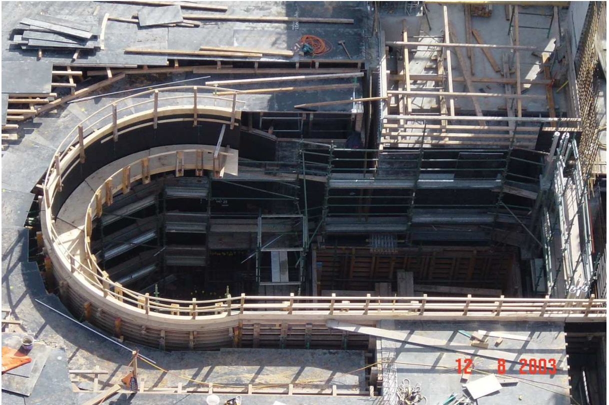
Replacement Research Reactor, Lucas Heights NSW: Image provided by the Australian Nuclear Science and Technology Organisation (ANSTO)
